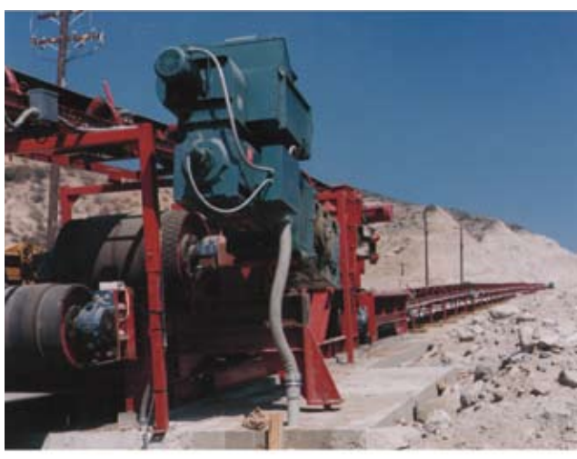
Figure 10. (Please provide a caption). Photo Courtesy Continental Crushing and Conveying
